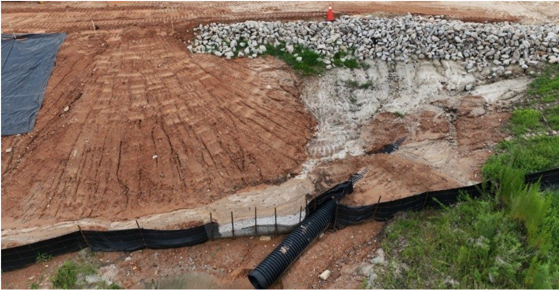
Erosion-control detail — silt fencing, outlet pipe and rip-rap as installed, photographed at low altitude.
