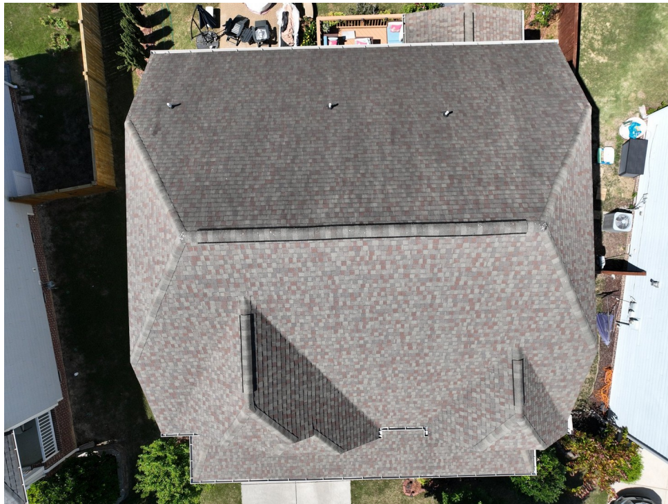
Fig. 1 — Full-roof overhead: hip-and-gable configuration, uniform shingle coverage, continuous ridge line with ridge vent, three plumbing vent stacks on the rear slope.
