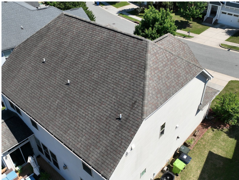
Fig. 2 — Oblique, street side: main and wing slopes in context; ridge and hip lines straight, gutter line continuous, no displaced material visible on any slope in frame.
