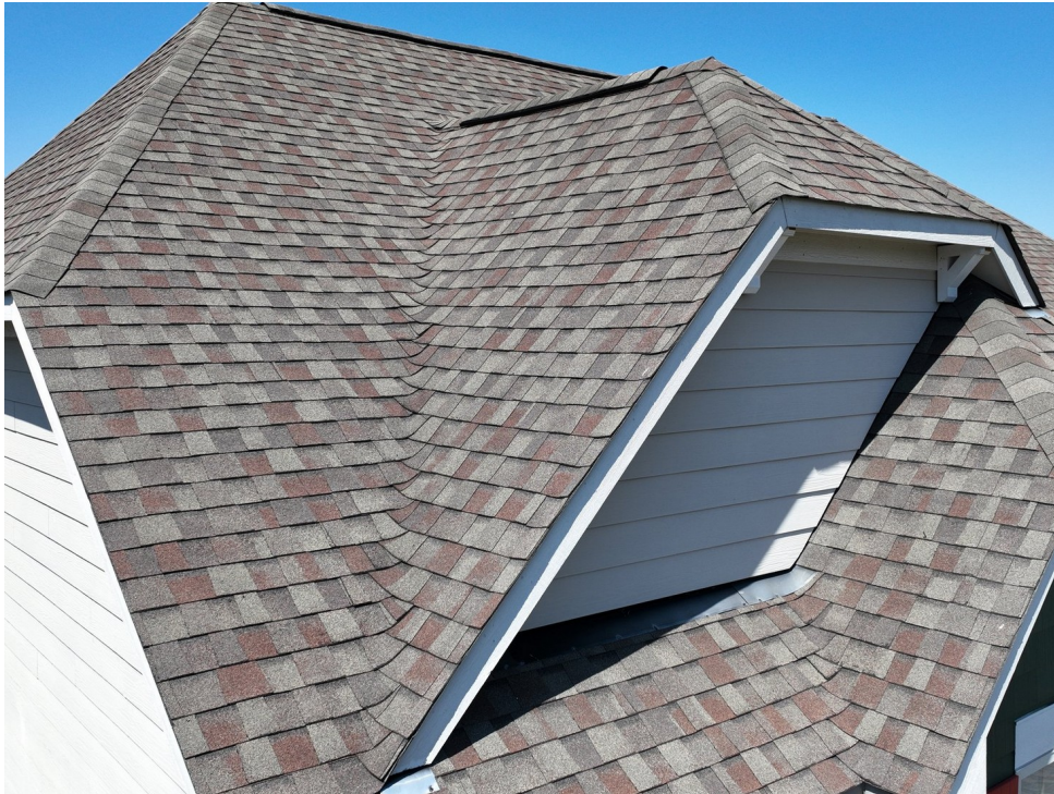
Fig. 3 — Oblique, dormer and upper slopes: valley and hip intersections seated, dormer flashing lines visible and continuous at capture resolution.
